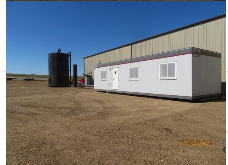
Soda Lake Facility – July 2025
